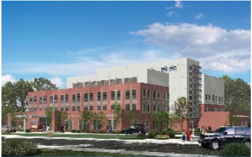
Sorg & Associates: US Embassy in Kathmandu, Nepal
